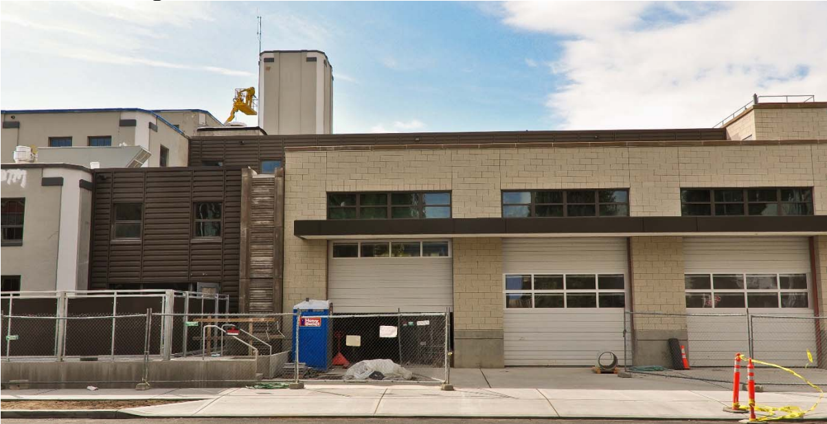
Station 17 Under Construction April 2010 Bob Lukas Photo
