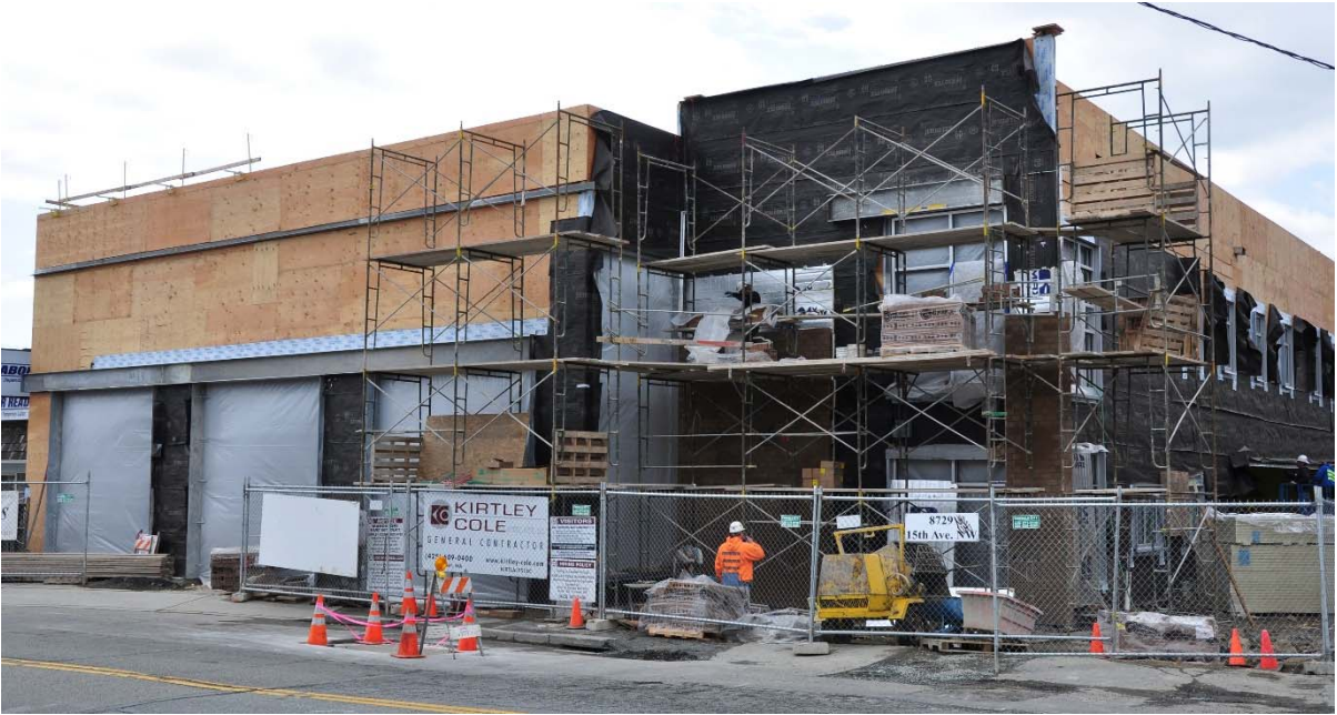
Sta 35 Under Construction April 2010 Bob Lukas Photo
